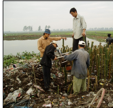
Figure 3 : Construction of Soil Conditioning Plant
