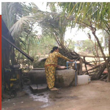
Figure 4: This pipe is Connecting Water from the Project
