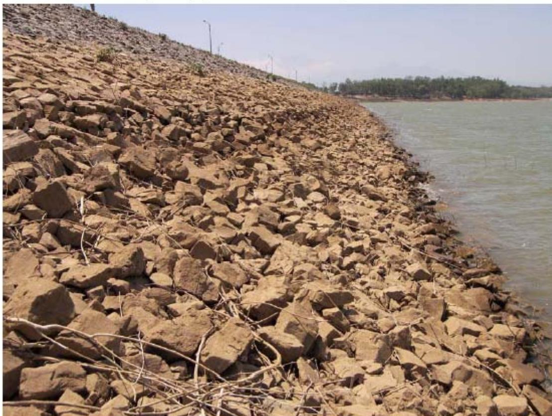
A10: Wonogiri Dam; Upstream slope with wave erosion scars
