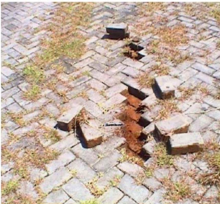
**A18: Parangjoho Dam, Crack underneath tiles on dam crest**
