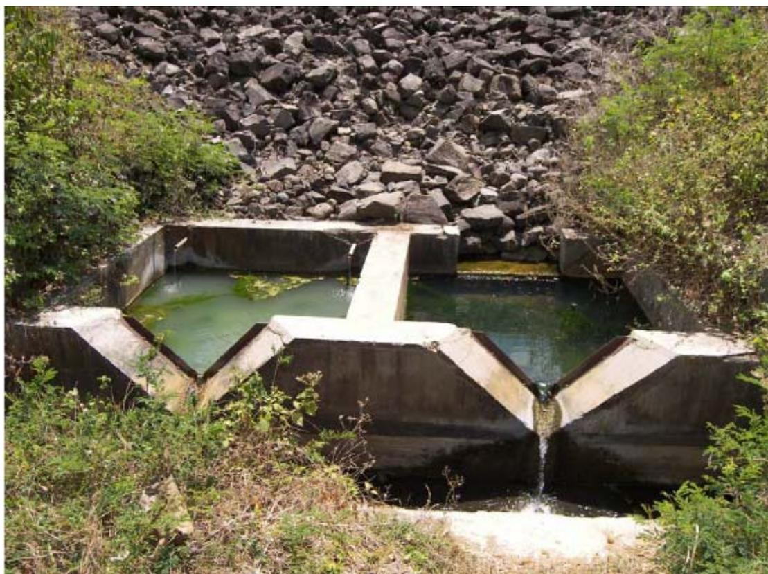
A21: Parangjoho Dam, Dual seepage measurement weir
