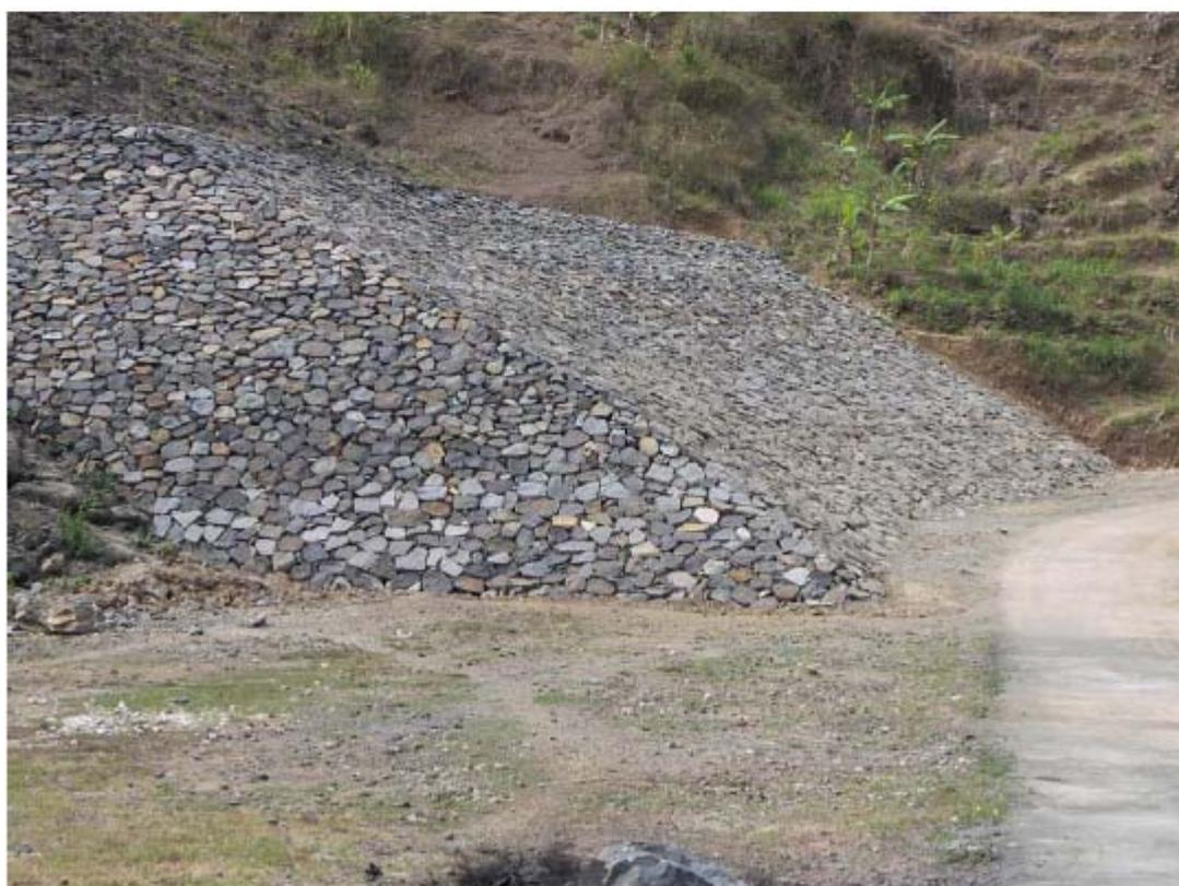
**A6: Sermo Dam; Buttress fill in the toe at the left abutment**
