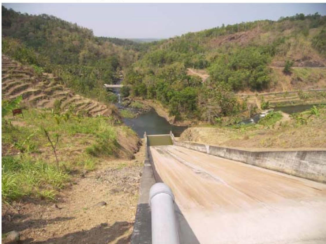
**A4: Sermo Dam; Spillway release channel and flip bucket**
