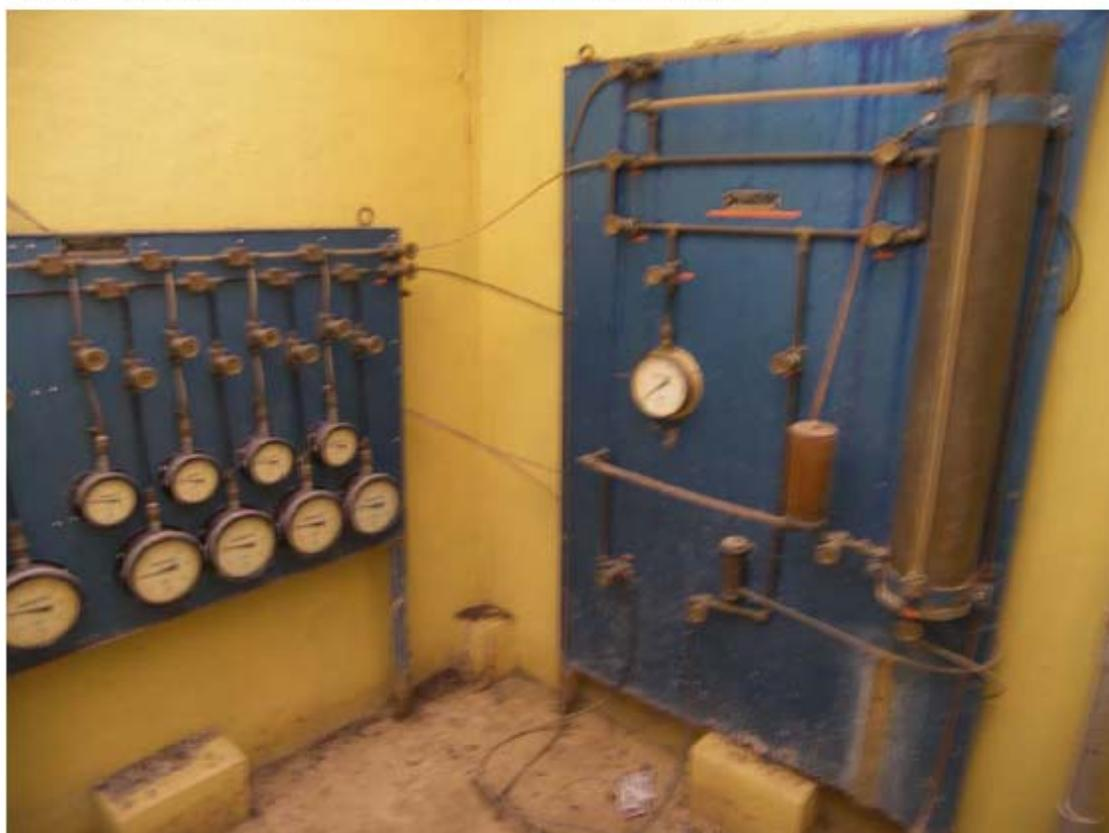
A22: Parangjoho Dam, Hydraulic piezometers
