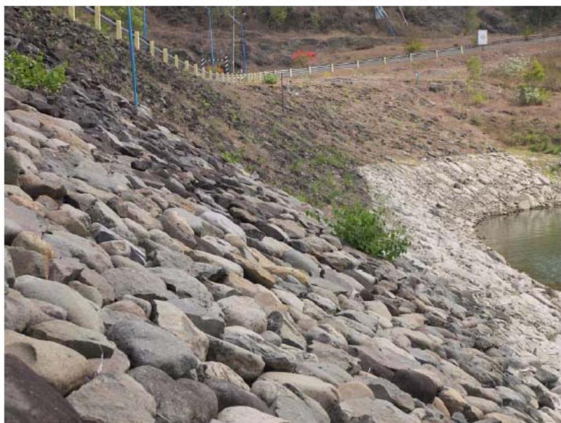
**A2: Sermo Dam; Rehabilitated and original riprap at right abutment**
