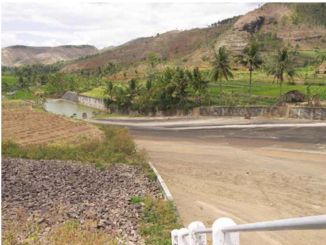
**A20: Parangjoho Dam; Spillway channel and energy dissipator**
