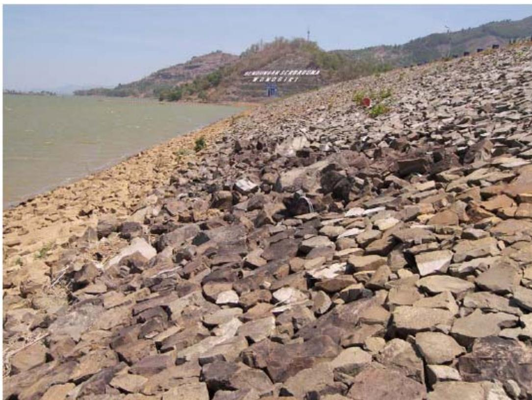
A13: Wonogiri Dam; Upstream slope; Newly rehabilitated riprap possibly displaced during earthquake shaking
