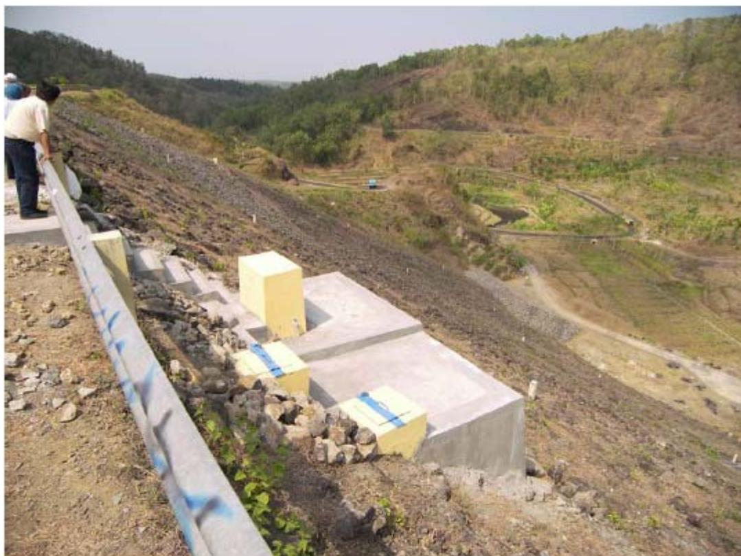
**A5: Sermo Dam; Downstream slope; Instrument installation in the foreground; Buttress fill in the toe at the left abutment**
