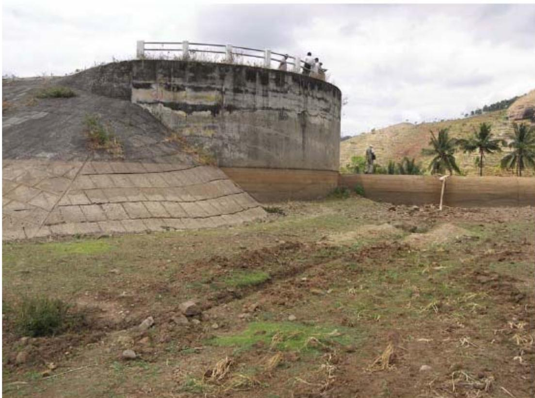
**A19: Parangjoho Dam; Spillway approach channel and fixed crest**
