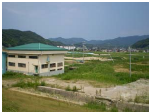
Balancing different land-uses such as agricultural lands, housing, infrastructure (for example, the pump house above), and residential housing (in the background) is a critical objective to sustain the economic growth of Toyooka.
